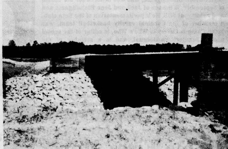
This county bridge on Martin Creek at the fourth and fifth district line was damaged by December 1982 flooding and repaired with a Soil Conservation Service grant of $16,135.80 through the Emergency Watershed Protection (EWP) program. The county experienced three major floods between December 1982 and May 1983 that caused over two million dollars in damages to farmland, drainage systems, conservation structures, and roads and bridges.
