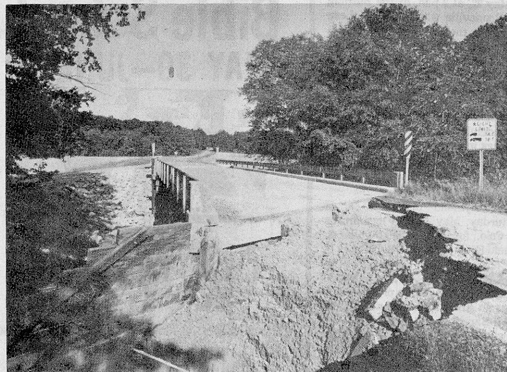
WASHOUT — This bridge across state-maintained Highway 366 is symbolic of the damage suffered by area roads as a result of rains this spring. Some roads have already been repaired once, or more, only to wash out again during the next rain. (Photo by Tim Rowland)
