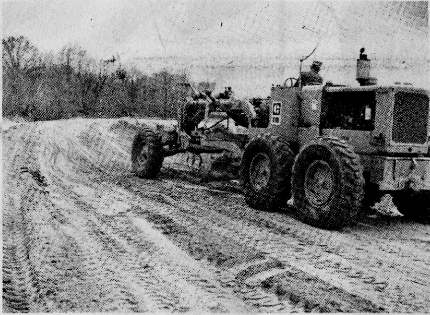
Leveling The Right Of Way
