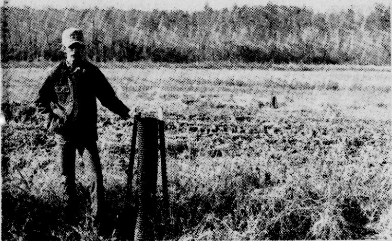
RONNIE BREEDLOVE looks over the parallel terrace system with pipe outlets he installed on his farm in the spring of 1980. Ronnie, like all other Prentiss county farmers who have installed the new terrace system, says he is well pleased with the results. During the year a total of 52,800 feet of terraces and 4,690 feet of underground pipe outlets was installed to help reduce soil erosion on sloping cropland. A total of 1,372 acres of cropland was adequately protected through the application of conservation measures in 1980.
