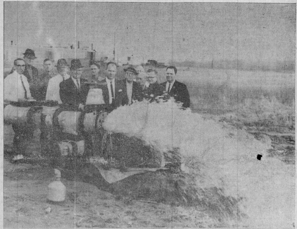
543 GALLONS PER MINUTE—City officials inspected the new water well Wednesday at noon prior to acceptance of the job from the contractors. At the end of the 24-hour test period Wednesday it is still pumping at the rate of 543 gallons per minute. Left to right are Leland B. Cook of Cook, Coggin, Kelly and Cook, consulting engineers, Tupelo; Jim Scott, superintendent of the water system until his recent retirement; Bob Herndon and J. H. Homan, Sr., Herndon and Homan Well & Supply Co., Inc., Shannon; Mayor M. W. Smith; T. B. Harris, acting superintendent; Aldermen Charles Steen, John Mahaffy and E. T. (Rob) Sartin; O. J. Robertson city clerk; and Aldermen Lealon George and Charles Crabb.
